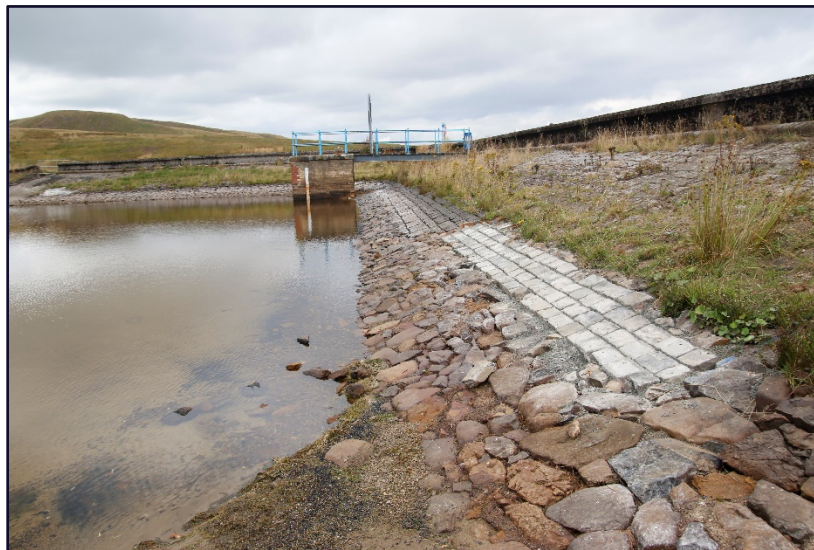
Fig.4. Reclaimed whin setts on east facing wall
