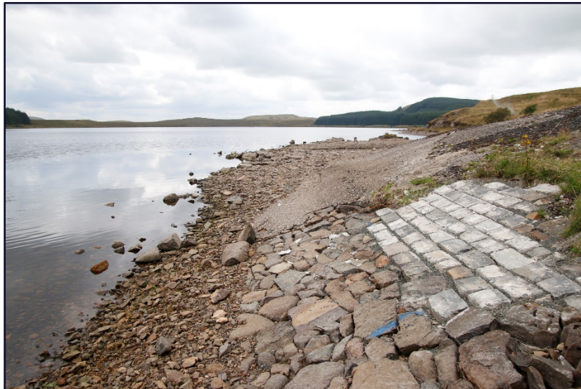
Fig 6. Reclaimed setts on north facing wall west of spillway entrance
