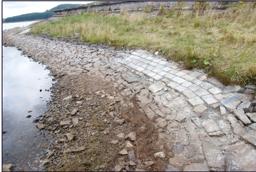
Fig 5. Reclaimed whin setts on North facing wall
