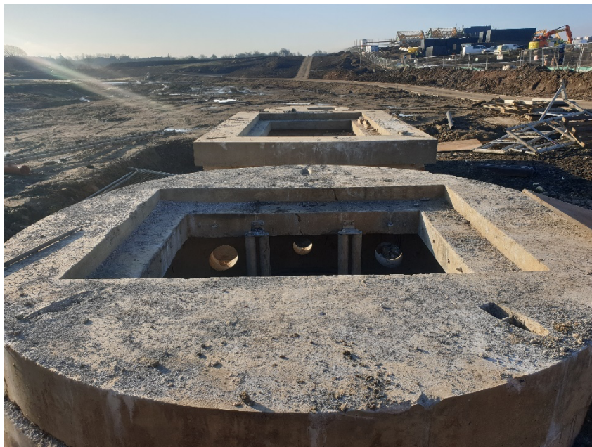
Fig10. Cover slab set to correct orientation and pump guiderails installed.
