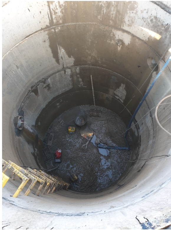
Fig.8 Surplus concrete to be broken out.
