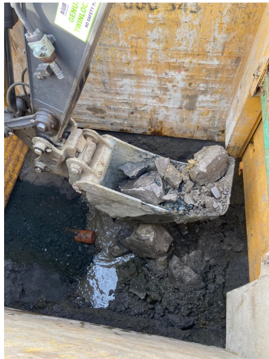
Fig. 6 Rock being removed from Excavation.
