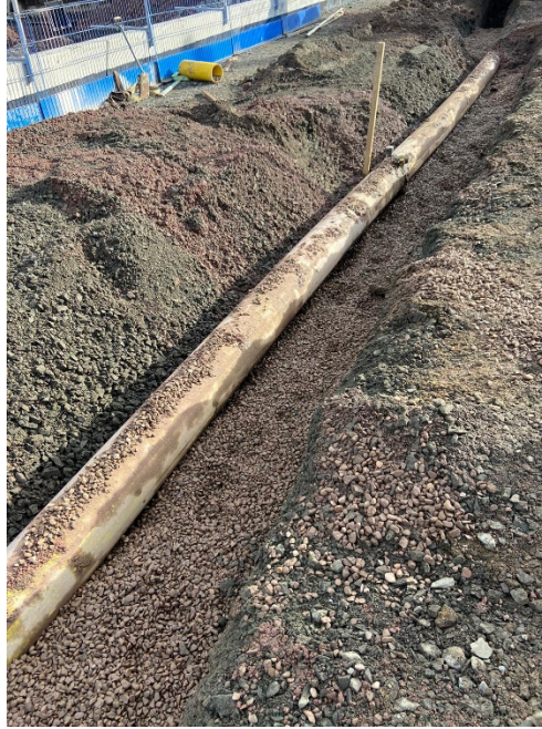
Fig.2 Medium Pressure Gas Main within excavation.
