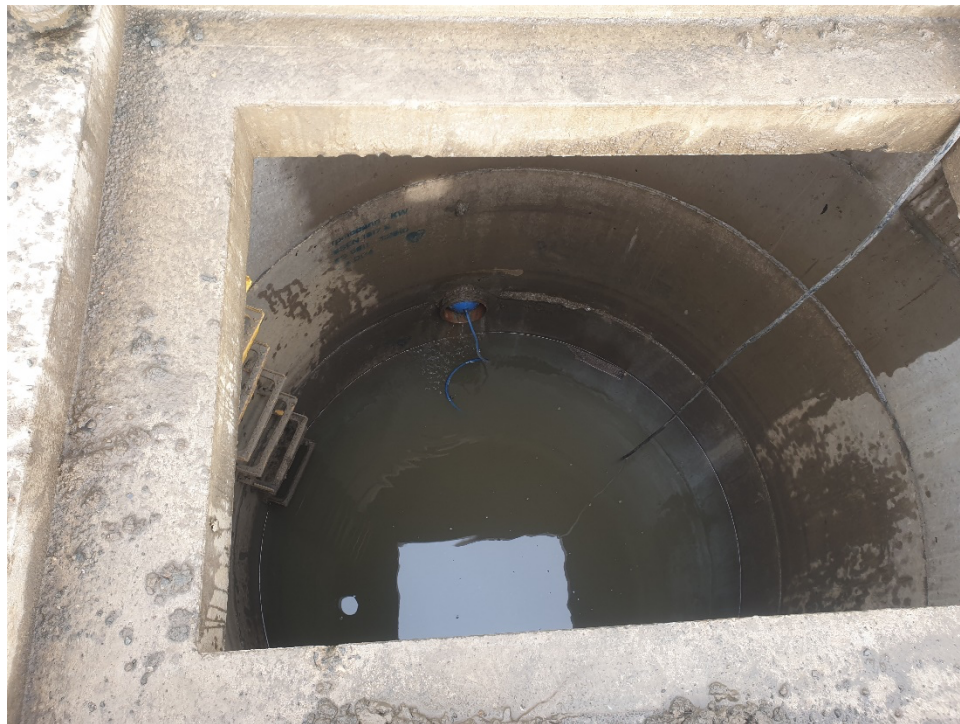
Fig. 7 Water ingress from underside of inlet pipe despite inflatable stopper being in place.
