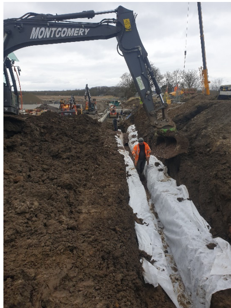
Fig.3 Laying bedding prior to pipe installation.
