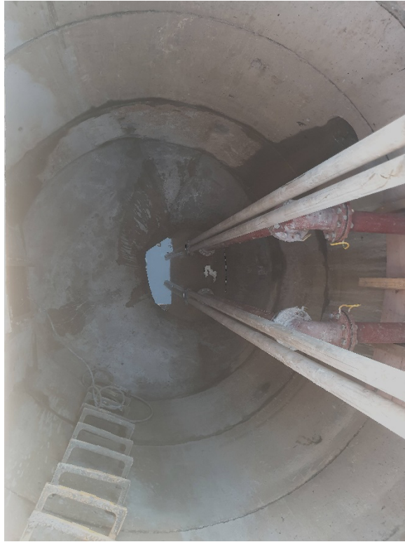
Fig. 9 Granolithic benching complete and pipe work installed.
