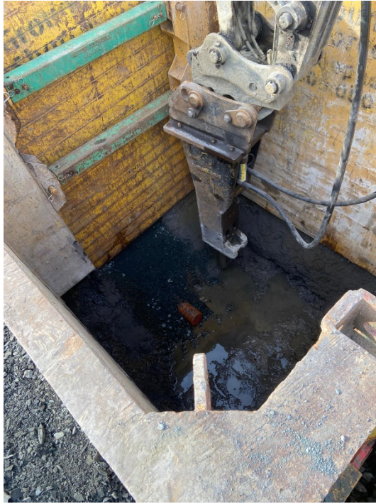
Fig.5 Pecker Attachment used to Break out rock.
